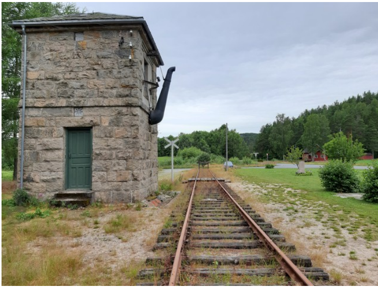
The water tower seen from another angle.
