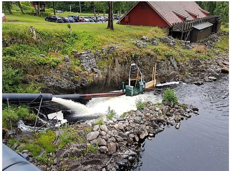
Below the bridge there is an overflow pipe.
