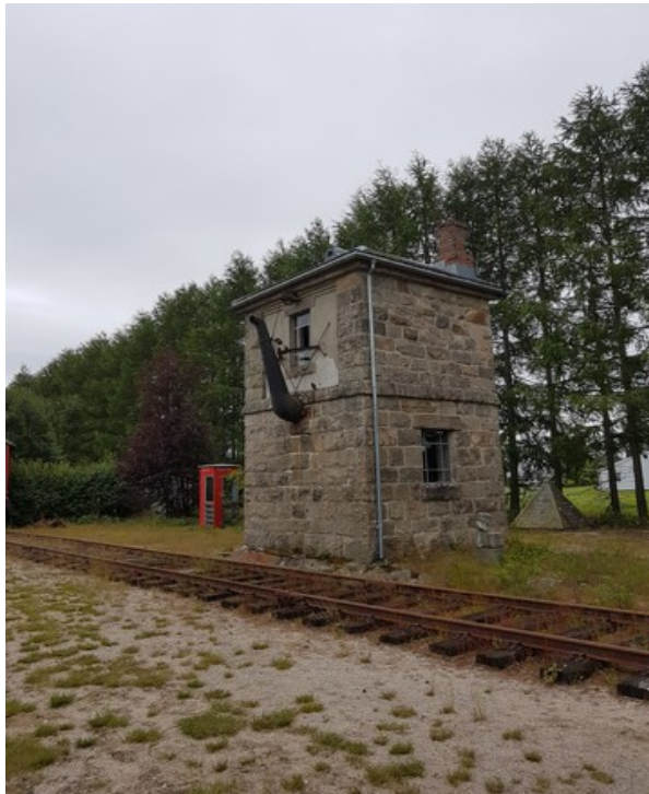
This water tower stands by the railway line at Simonstad station on the Treungen line . Here you could fill the steam locomotive with water. The railway line ran between Arendal and Treungen .
