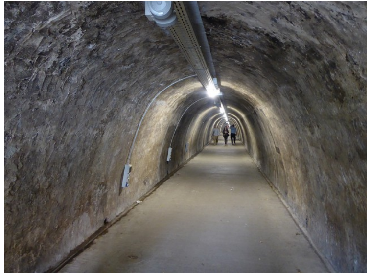
This is inside the tunnel.
