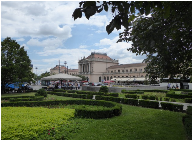
Zagreb Glavni kolodvor , the main railway station was opened in 1892.
