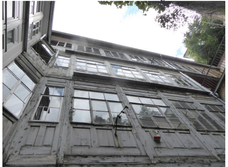
This entrance is in a courtyard of a building with very worn wooden clapboards.
