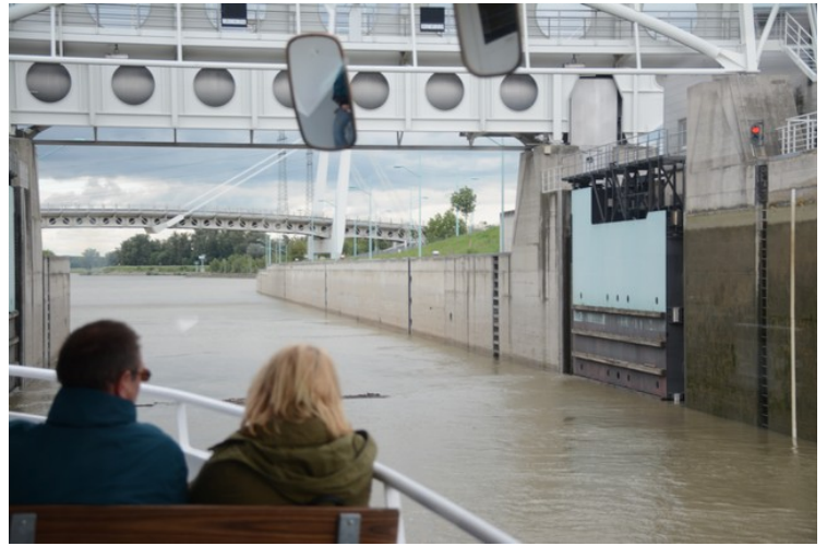
The lock gates are open and the boat can run out of the lock.
