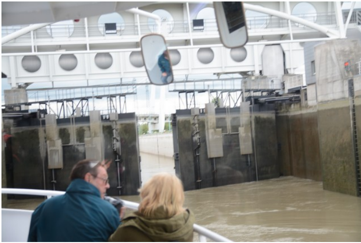
The water is out and the lower gates open.
