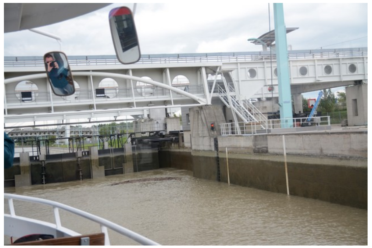
Draining water out of the locks has begun.
