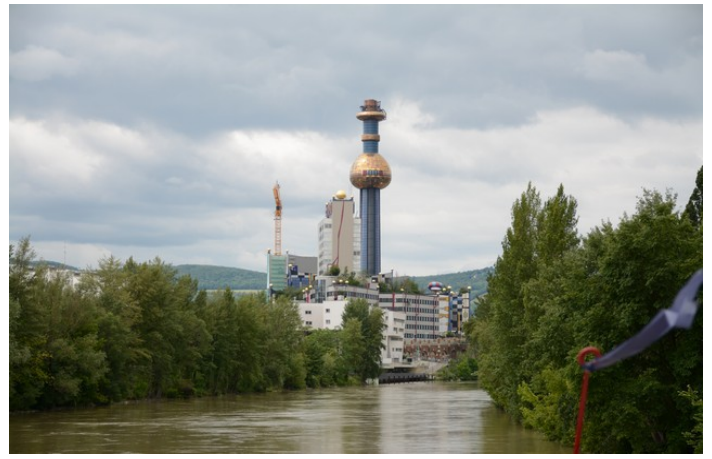
District heating plant Spittelau.
