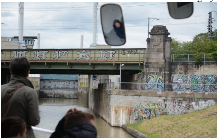
Into the first lock.
