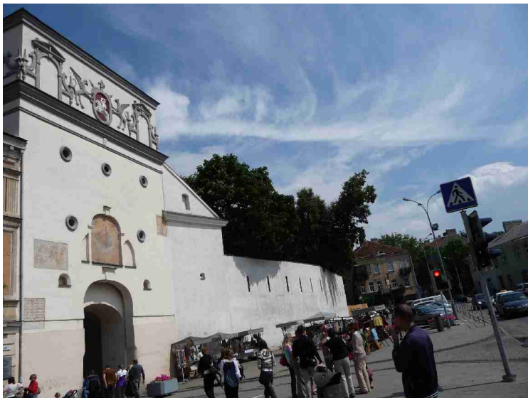
The gate looks like this on the other side
