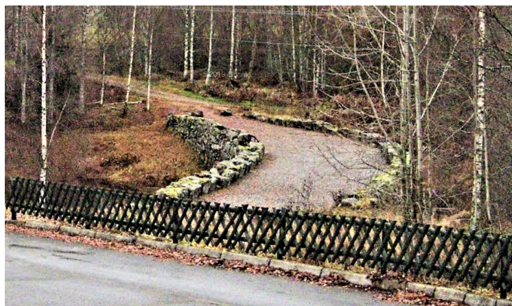
Right beside is this bridge where there once was a road.
