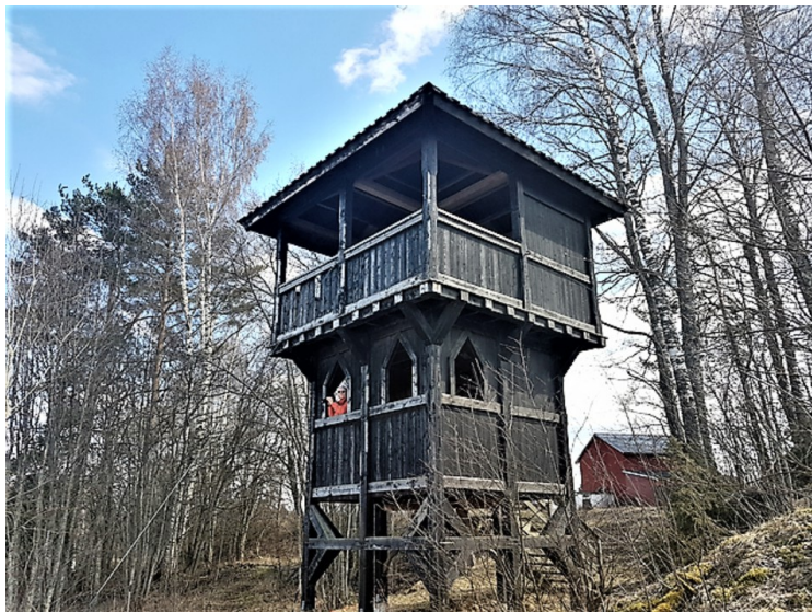
The tower seen from below.
