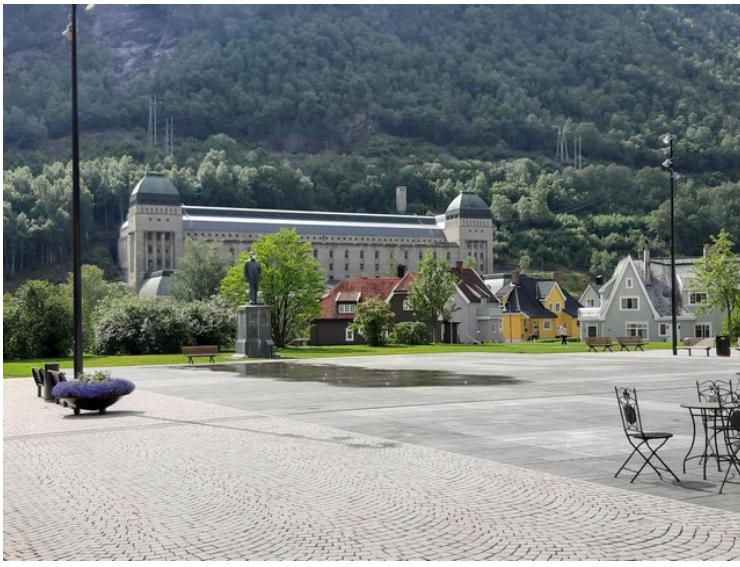
Såheim power plant was put into operation in 1916.
