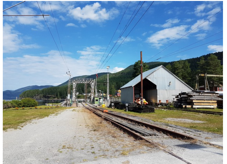
Here is the terminal and slipway to be able to inspect the ferries.
