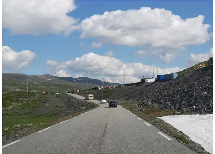
The Haukeli tunnel has the eastern opening on the right.
