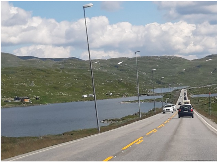
This is Ståvatn .
