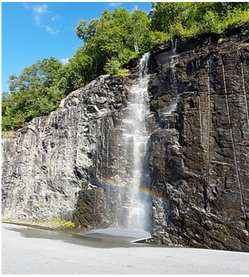
Here comes the water that will make the waterfall on the viewing platform.
