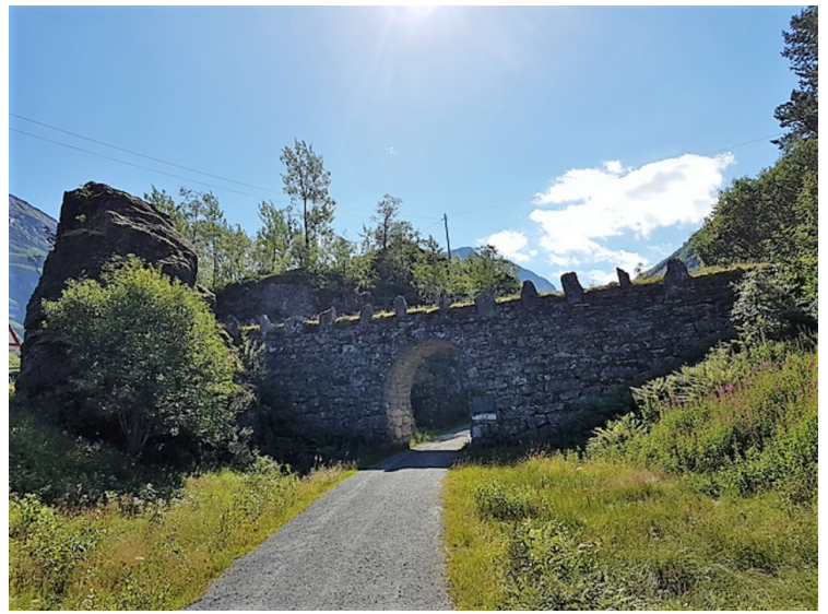
We stopped at Knuten . It was constructed when Geirangervegen was built, to overcome height differences in difficult terrain.
