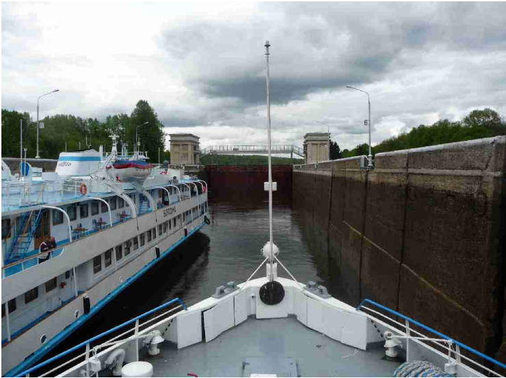
Most of the water is drained.
