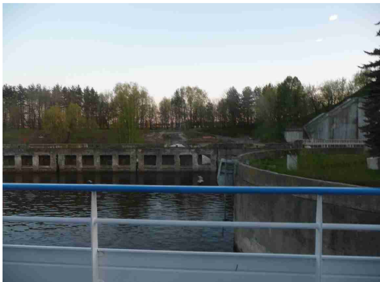
Here we are down and out of the lock.
