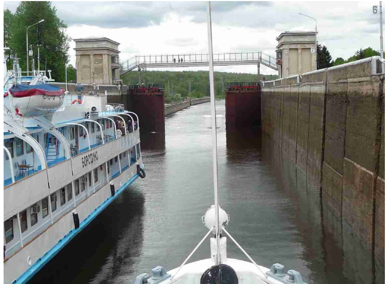
The lower lock gates are opening.
