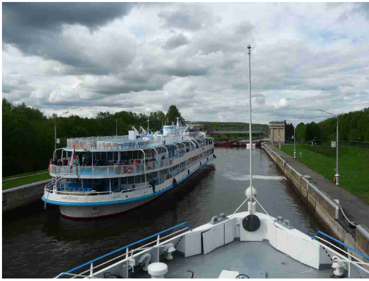
There is room for two ships in the lock. The length of the locks is 290m and the width is 30m.
