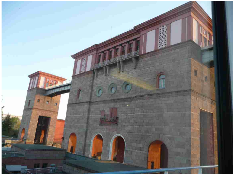
This is a double lock. Boats can be sluiced upwards and downwards simultaneously. It is the last lock before arriving at Yaroslavl.
