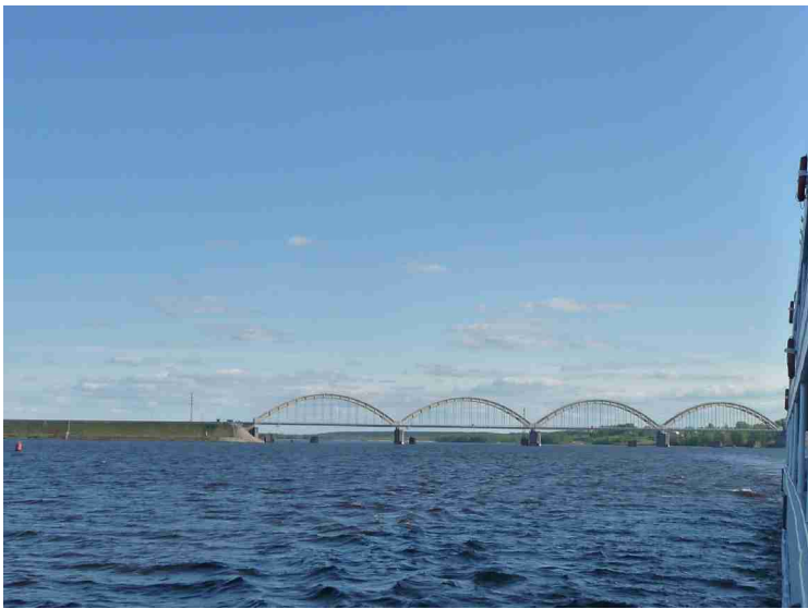
A large railway bridge cross Volga here.
