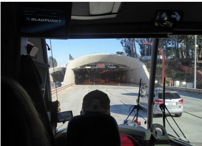
At the end of the bridge there is a short tunnel.
