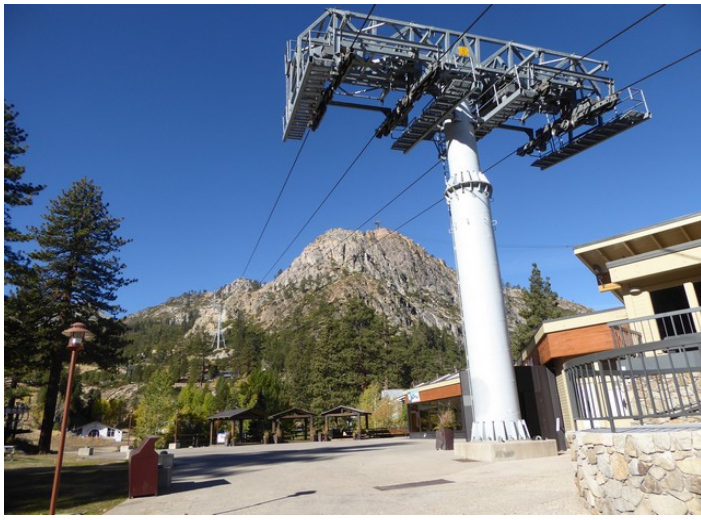
One of the mast for the ski lift downhill.
