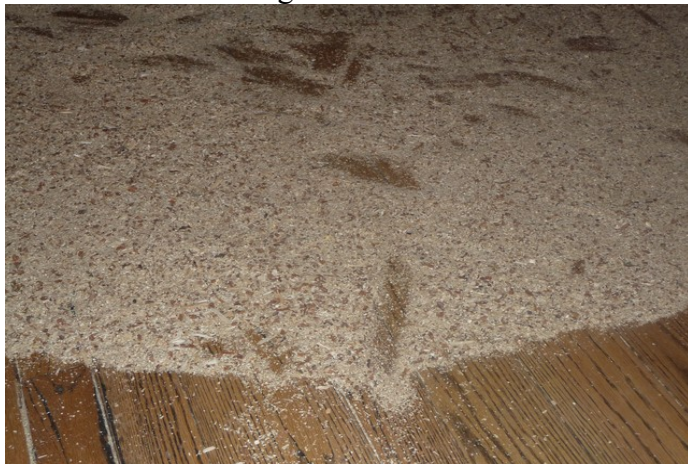
Sawdust on the floor.
