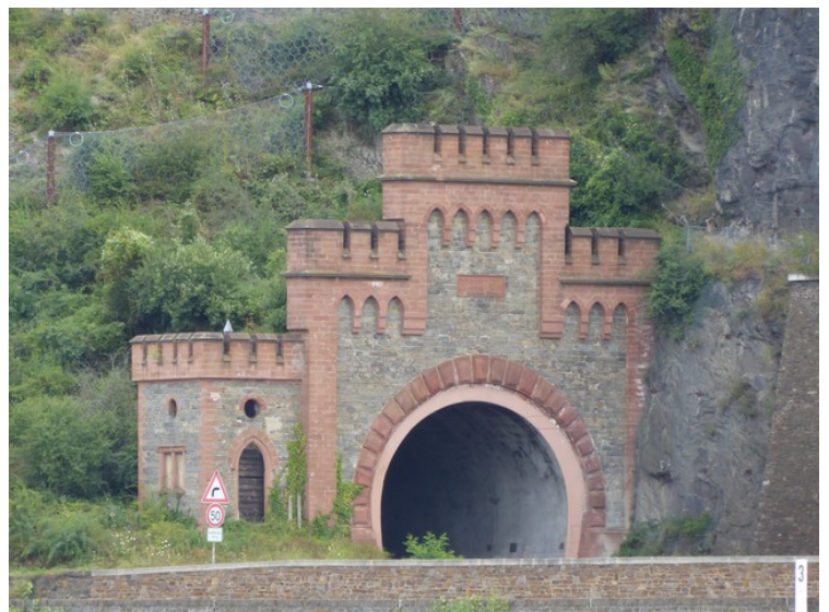
We look across the river on a railway tunnel.
