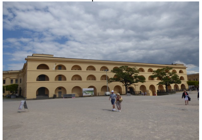
This building is part of a ring wall.
