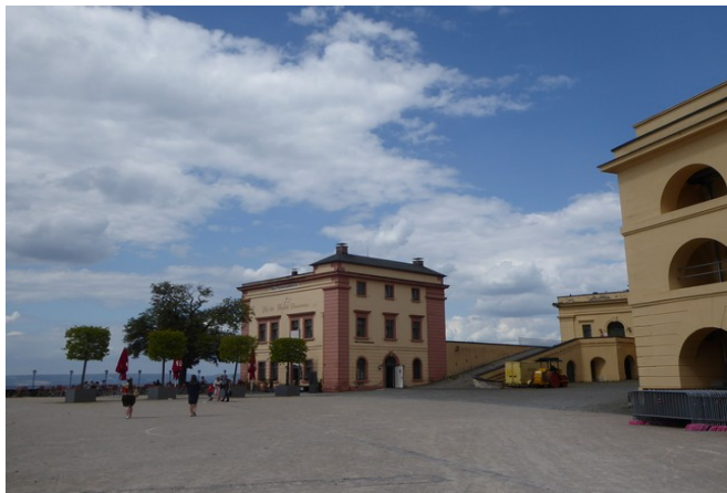
The upper castle square (Obere Schlosshof). The house straight forward is a restaurant today.
