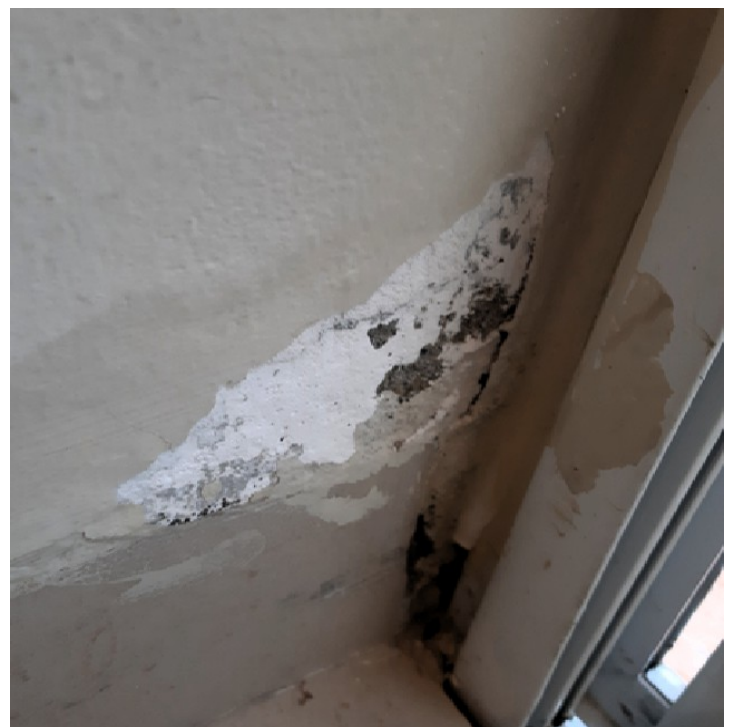
One of the shortcomings was plaster that had loosened from the wall in some places.
