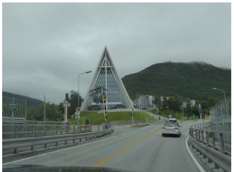
There were different things we wanted to see in Tromsø, but there was so much road work going on and poor accessibility that we got tired and just drove on. Here we are on the Tromsø Bridge on our way back to the mainland. The Arctic Cathedral straight ahead.
