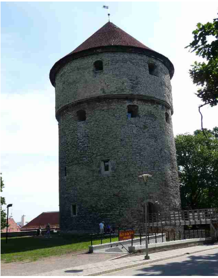
On our way into the town the first day, we have reached Kiek in de Kök. It was built as a cannon tower late in 1475. The tower is 49,4 meter high, has a diameter of 17 m, and the walls are 3-4 m thick. It was once the largest of its kind in North Europe.
