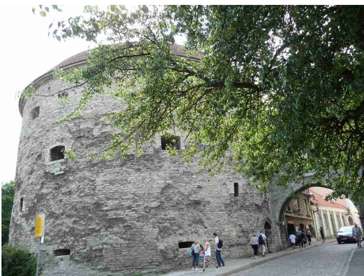
The tower Thick Margareta. It has a diameter of 25 meter and the walls are up to 5 m thick.
