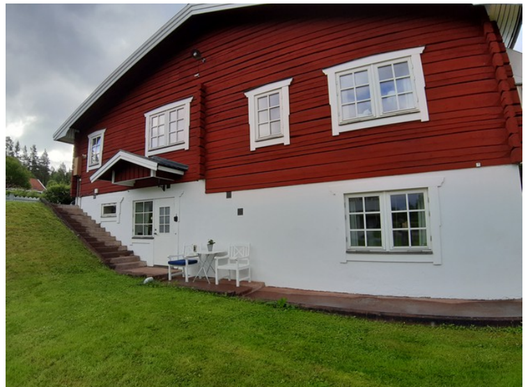
We had to go down a flight of stairs to get to the entrance of the apartment we had rented.
