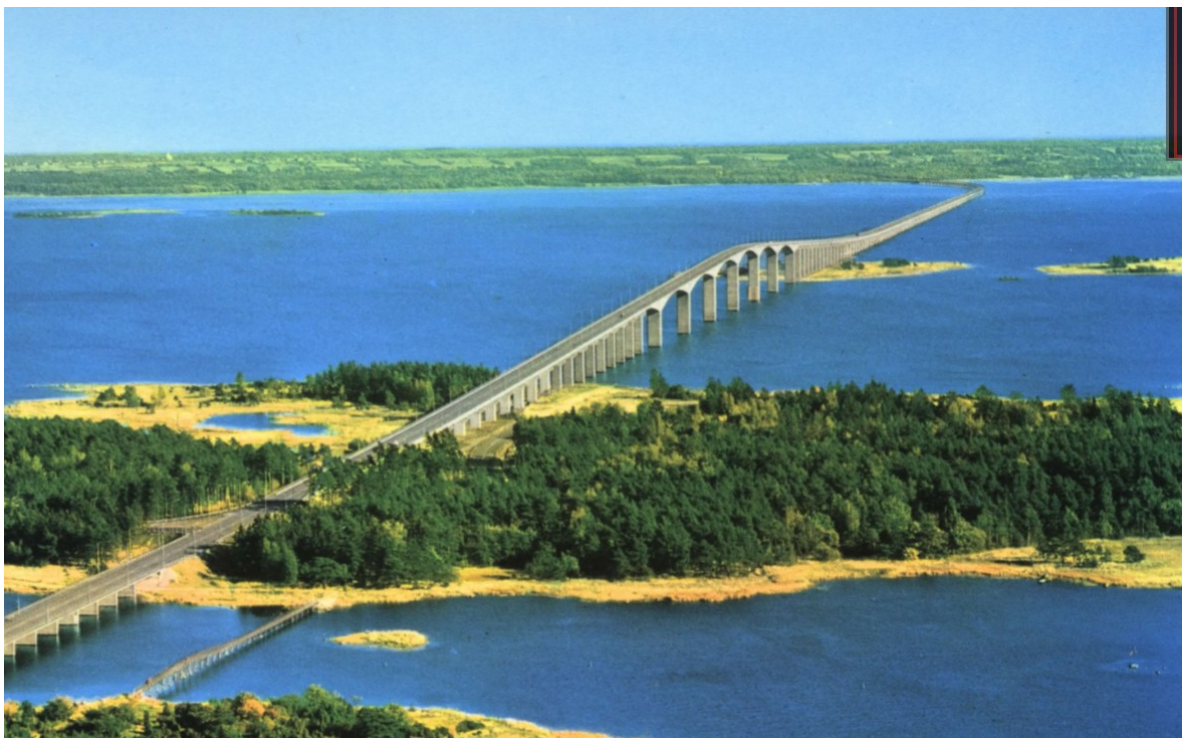
Ölandsbroen is the longest car bridge in Sweden, 6,072 meters long, clear height is 36 meters. The bridge is built in reinforced concrete in 155 spans, the highest part has 6 spans with a span of 130 metres. It connects Öland with the mainland at Kalmar. It was opened in 1972, and for several years was Europe's longest bridge.
