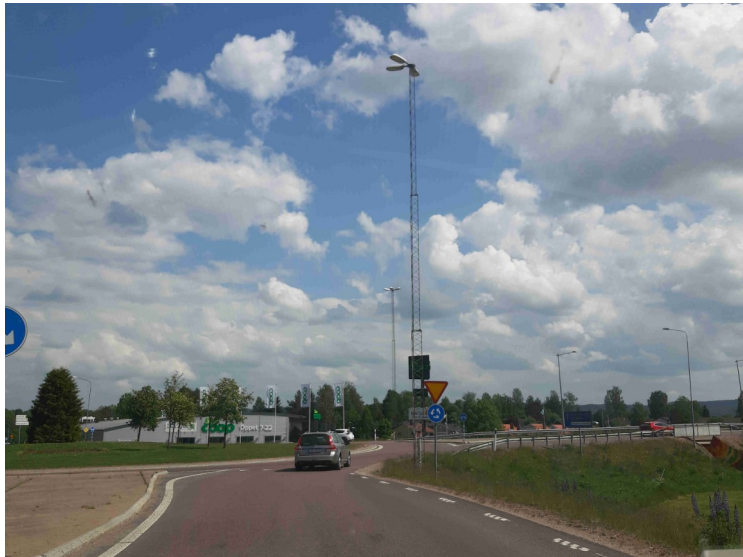
The roundabout at the junction between E16 and E45.
