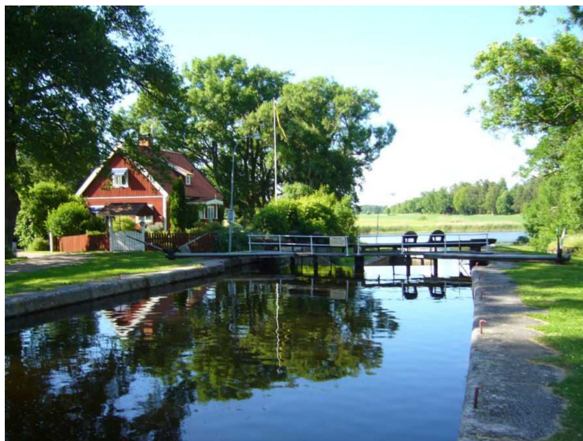
The Gravudden locks are two manually operated locks along the Hjälmare canal, They are located just outside Arboga. The locks connect Arbogaån with Hjälmare and are the northernmost start or end point for Sweden's oldest still navigable canal. There are 9 locks in the canal. Via Arbogaån there is a further connection to Mälaren and the Baltic Sea.
