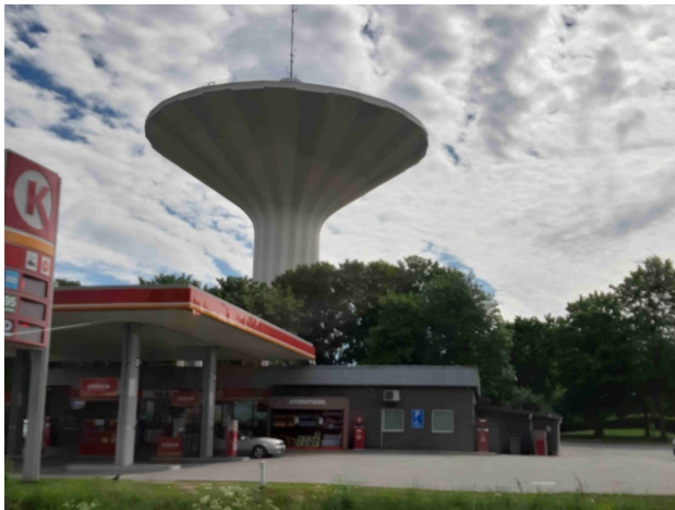
The water tower – Svampen (The sponge).
