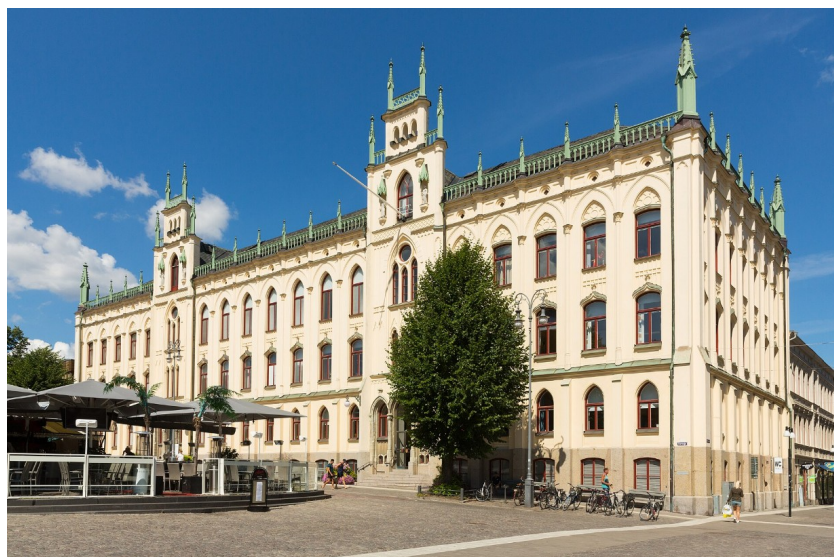
Örebro town hall from 1863 is located at Stortorget and is the seat of the municipality's political leadership and its administration.
