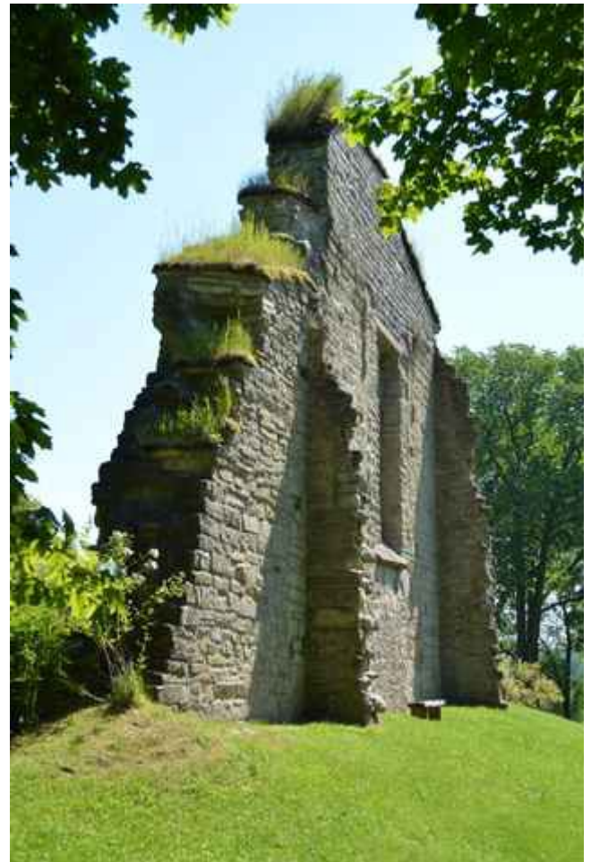
This wall is mostly what is left.
