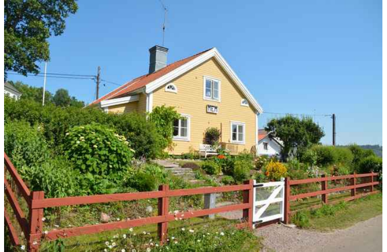
The lock keeper's house.
