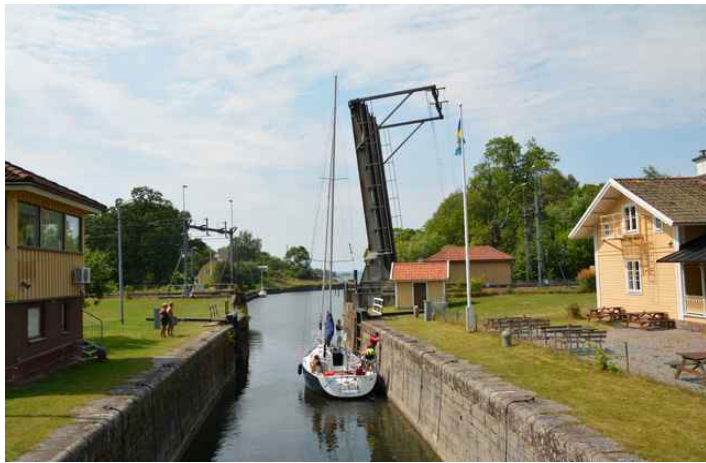
Here's a bridge that needs to be lifted up when a boat is going to pass.
