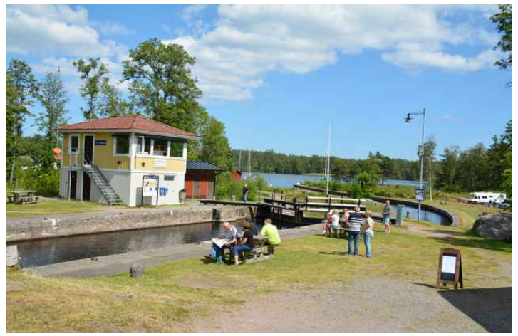
Forsvik . The highest altitude of the canal. 91.8 meter above sea level.
