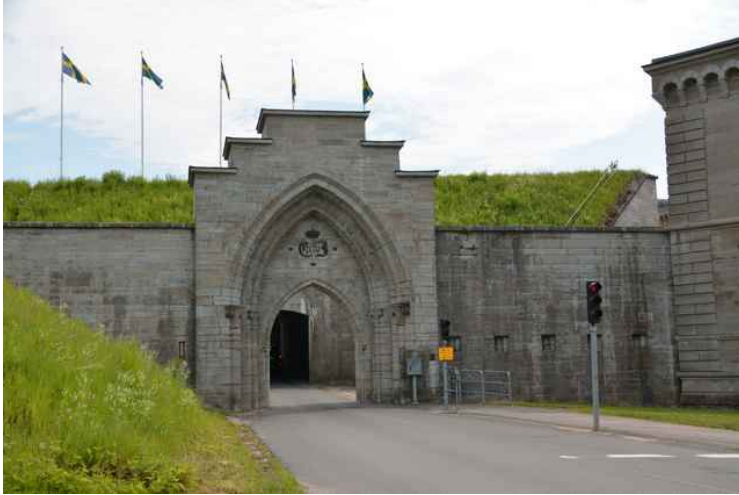
The main entrance with the Gothic gate (28).
