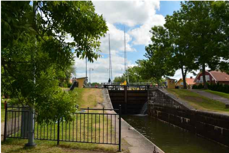
This is the lock that is located right on the main road through Sjötorp .
