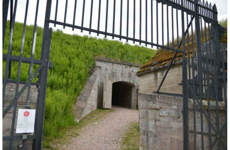
One of the entrances to Karlsborg Fortress .
