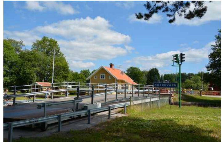
No lock, but a bridge that has to be lifted to let the boats pass by.
