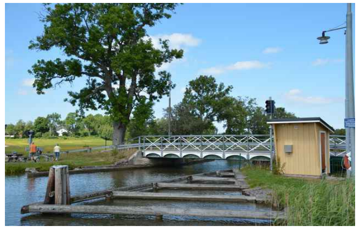
No lock, but a bridge that has to be lifted to let the boats pass by.
