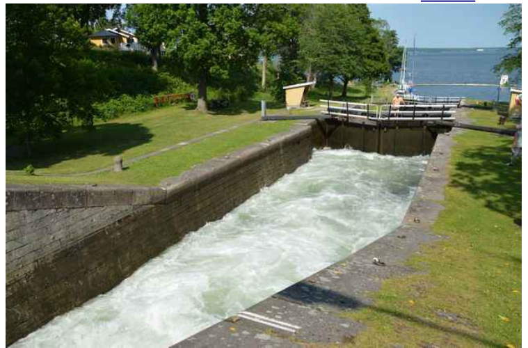
Quite a splashing in the lock chamber.
