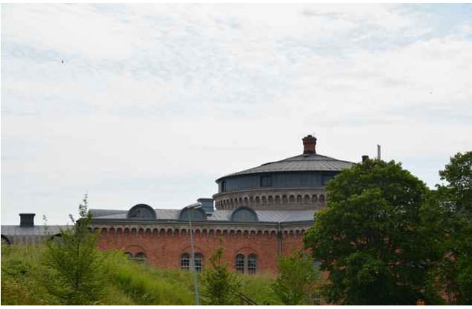
One of the three towers in Slutvänet (1), which is seen at the bottom of the picture. Slutvänet is Europe's longest heated building, 678m.
