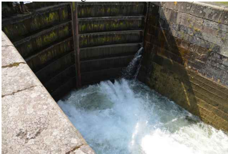
One of the lock valves is opened.
