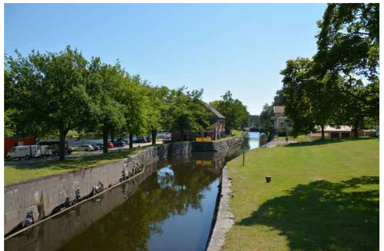
View from the bridge down the canal. The lock is farther away.
