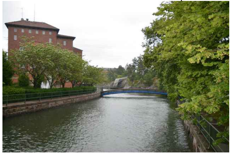
The canal leading down to Olidan power plants. It runs parallel to and between the Göta Canal and the Göta river.
