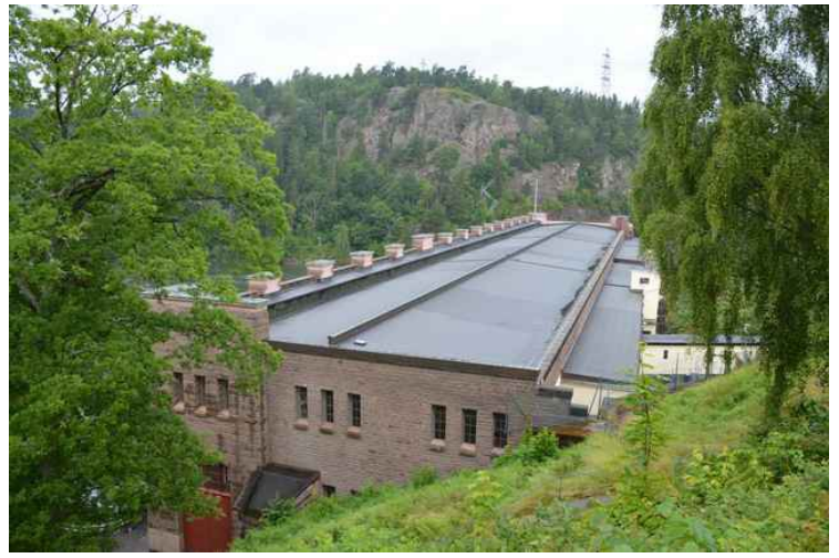
Olidan power station.
