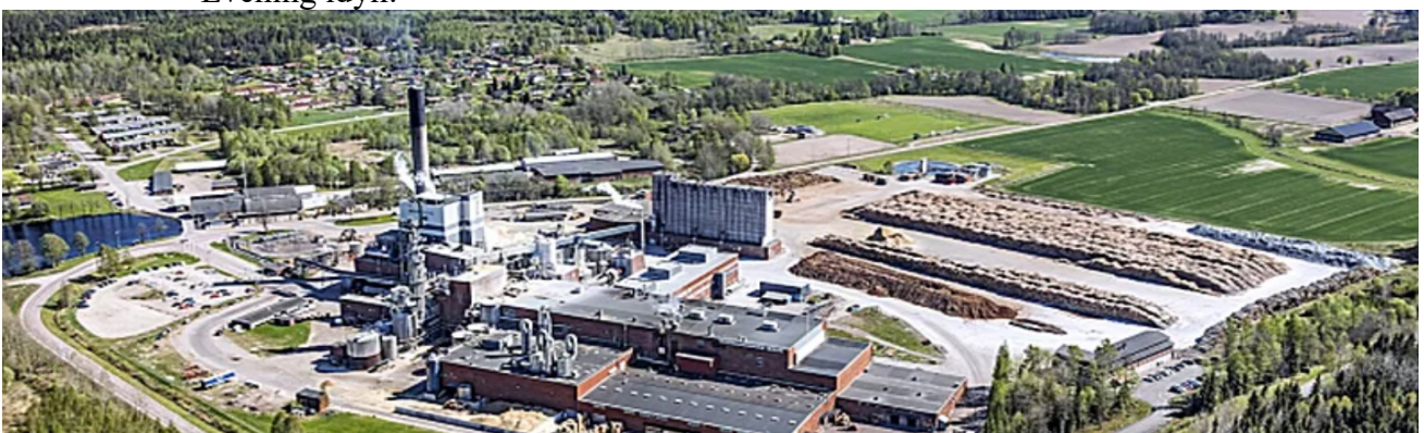
Areal view of Bäckhammar. The largest company is Nordic Paper .
