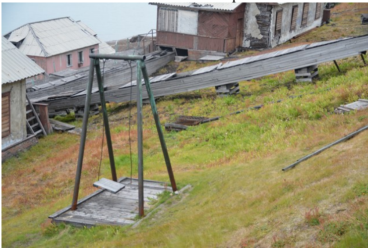
It does not seem that this is being used either.
