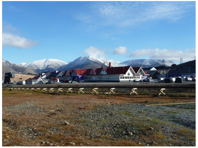
District heating pipes are laid in the bottom of the valley.
