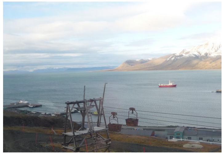
The same cableway with views along Adventfjorden towards Isfjorden.
