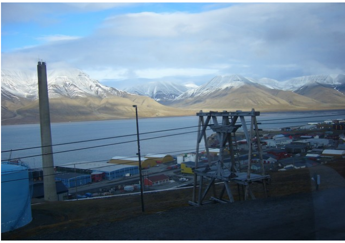
A portion of the cableway that goes to the coal pier. We see the chimney at the power station, Longyear Eneriverk , to the left in the image. The plant gets coal from Mine 7 , east of the village, and uses about a third of the 80 000 tonnes of coal annually broken in the mine.
