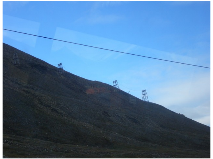
Cableway for the transportation of coal. It went from Mine 1 and down to the cableway center. It is not in use anymore.
