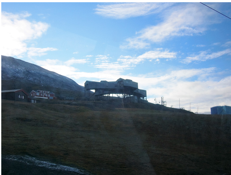
Three courses were collected in this Areal Ropeway Junction Building . It is now closed. The coal is now being transported by truck. It has been decided that it should be protected along with the cable car that goes from here to the coal pier.
