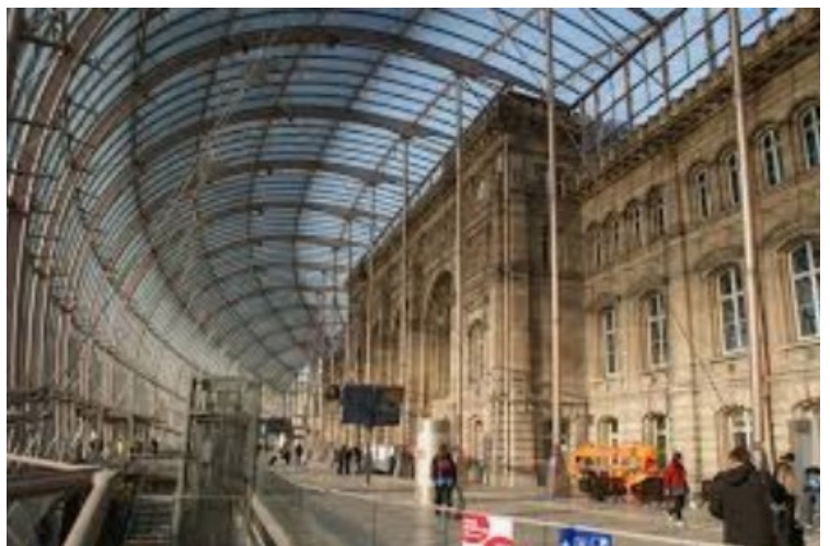
The facade with the glass roof above and in front.
