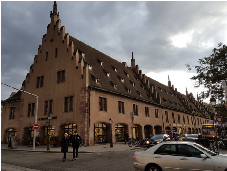
At the end of the bridge is the old customs house . It has been classified as a historical monument since 1948. It was severely damaged during the bombing at the end of World War II, but it has been restored.
