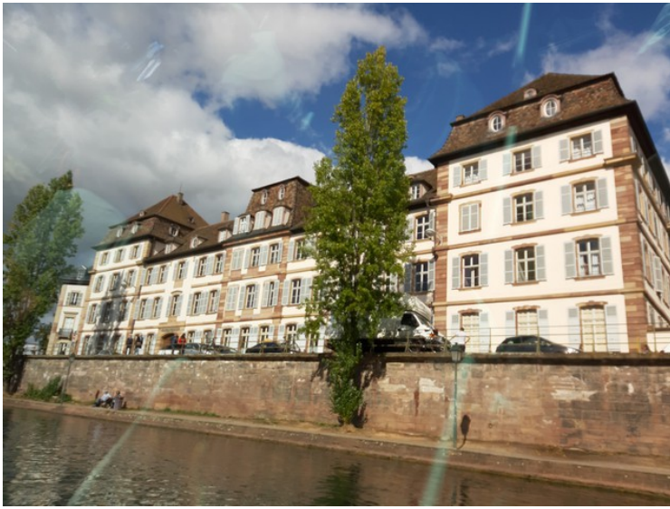
This building houses a protestant foundation, Le Stift .
