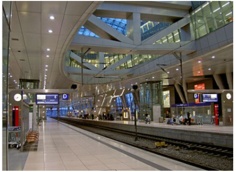
Inside the station.
