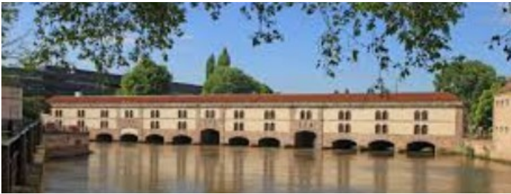
Barrage Vauban is a bridge, weir and defense works. It was built in the late 17th century. It should enable to raise the level of the River Ill and thus flood the area south of the city, to make it impassable for an enemy. This was done in 1870, when Strasbourg was besieged by Prussian forces during the Franco-Prussian war, and it resulted in the full flood of the northern part of the suburb of Neudorf.
