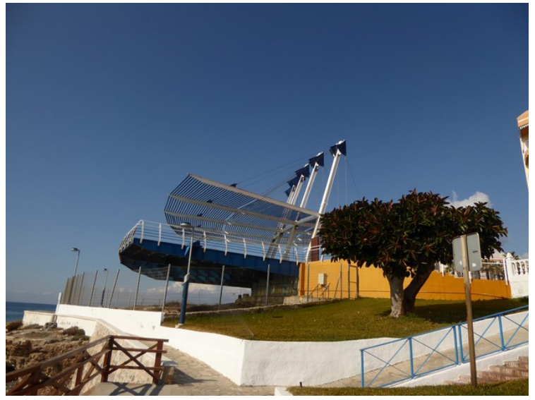
This is a balcony and viewpoint. Under the roof are ruins from a graveyard. About Torrox.
