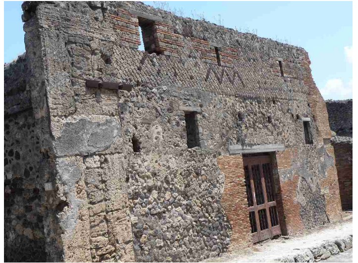
Another brick laying technique
