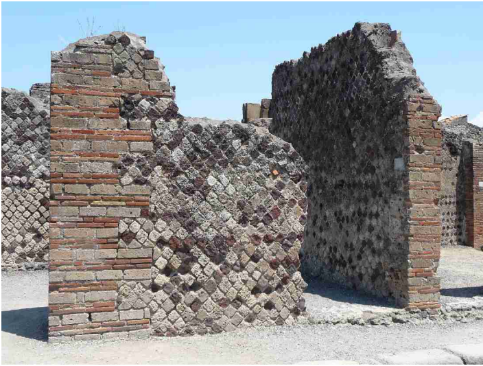
Various brick laying techniques
