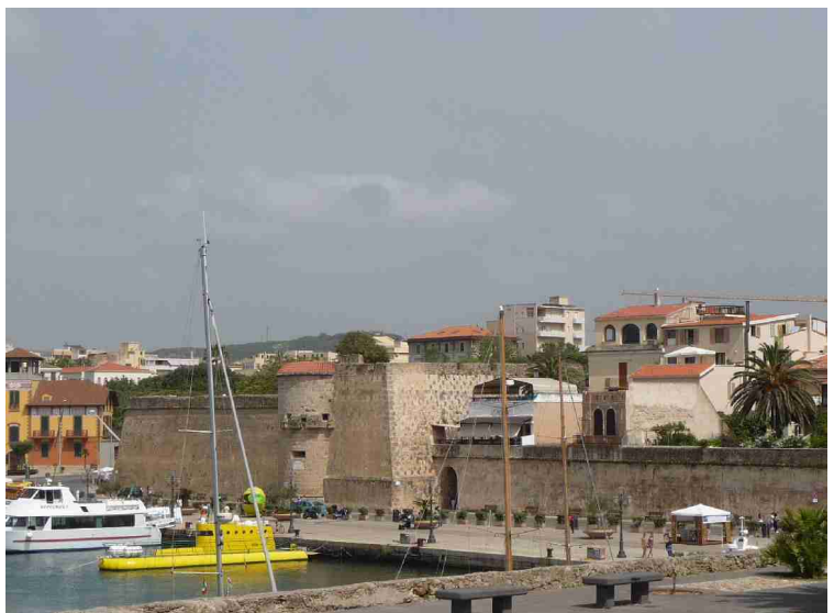
Here we are approaching the walls.
