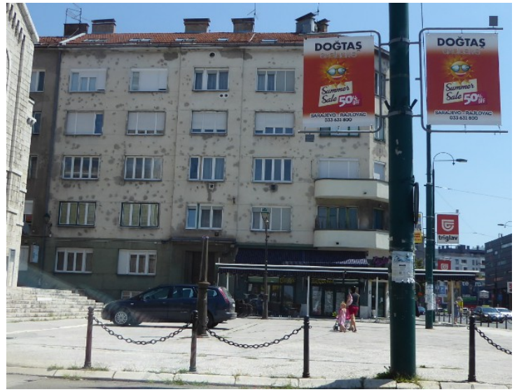
In this building there are still lots of bullet holes in the façade after the siege of the city in the 1990s.
