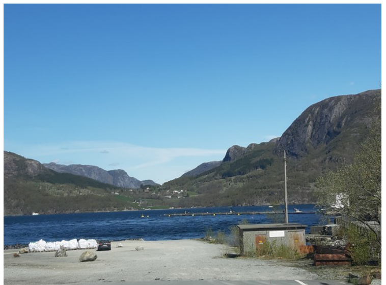
Then we were down by the quay in Oltesvik. Oltesvik Power Plant is located next to the quay. It gets water from Ragsvatnet, On the other side of Høgsfjorden we see Rossavik.
