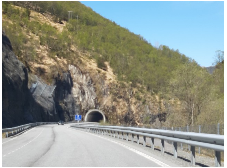
Then through this tunnel, the Skredlitunnel which opened in 2009. Before the tunnels opened, the road was narrow, winding and prone to landslides.
