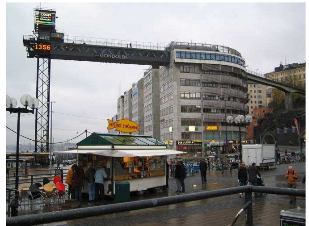
Katarinahissen ( an elevator ) was built the first time in 1883, because there are quite big differences in altitude on Södermalm. The last one was built in 1936.
