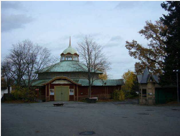
The Brage Hall. It was built in 1897 of the brewers in Stockholm for a fair this year. When the fair was over it was placed here. It is used for various arrangements.
