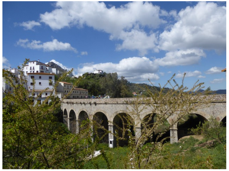
This is right before we come to the main road again. The main road goes on this viaduct.
