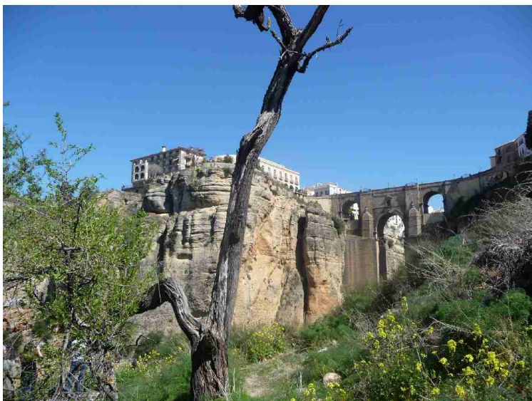
We are passing the gate and get a view up to the bridge.
