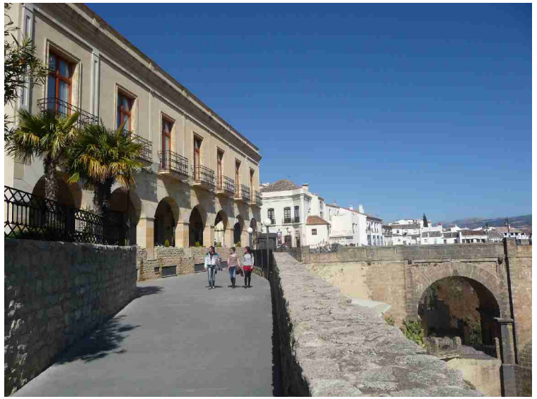
Looking the other way, towards the bridge.
