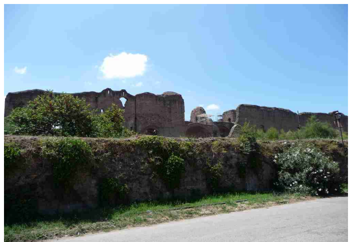
Here we are looking back in direction of the bathing facilities
