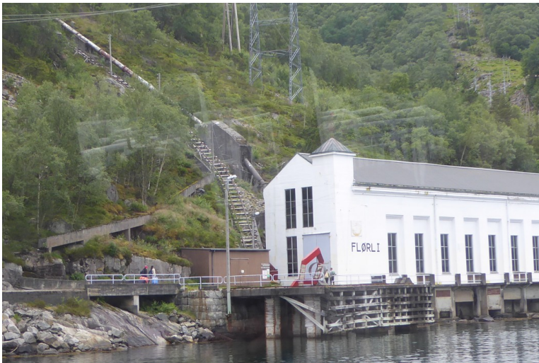
Here we see the lower part of the Flørlitrappene.
