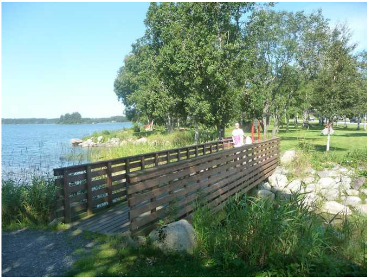
There is made a footbridge over the stream just before it flows into Frøylandsvatnet.
