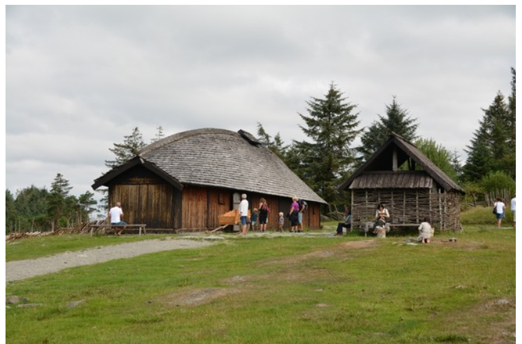
The long house on the left and the fire house on the right. The roof of the main house is covered with over 100,000 hand cut pine sheets.
