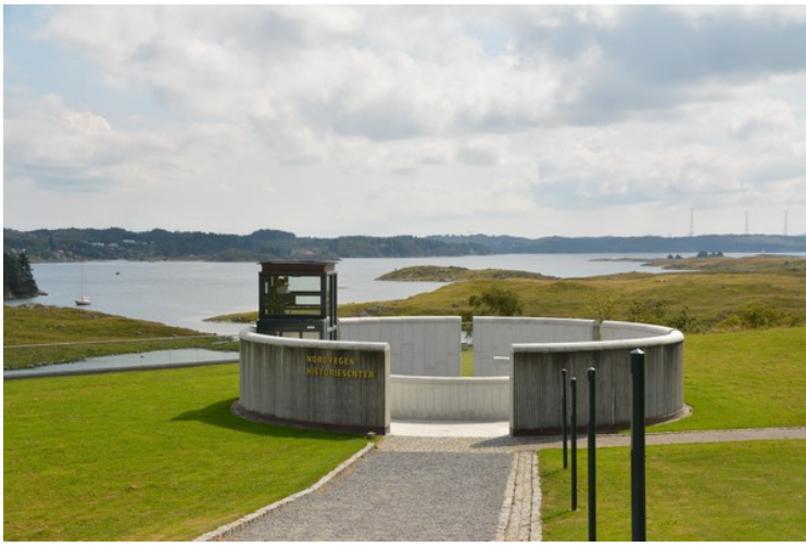
Right below the church lies Nordvegen History Centre . This is one of the windows in the roof.
