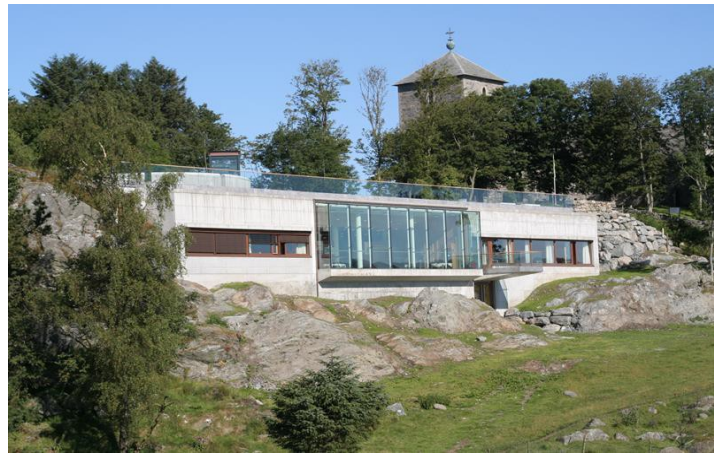
This is how it looks in the front. The plant is mainly buried in the ground so that it will not interfere with Olav's Church.
