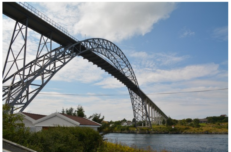
The are positioned right under Karmsund bridge.
