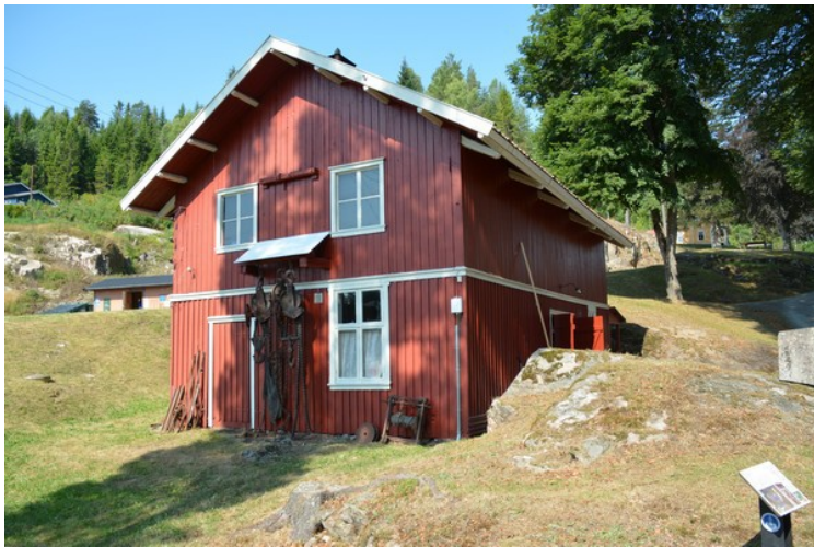
This is the forge. The forge in Vrangfoss was set up after the canal was built. It is built of material remaining after the construction period. Vrangfoss-smithy is the best equipped and most used smithy. Most of what was originally forged in the channel are maintained and repaired with forged parts. This applies, for example, railings, calipers and wear parts in the lock gates. In this way, the uniqueness of the channel is kept alive.
