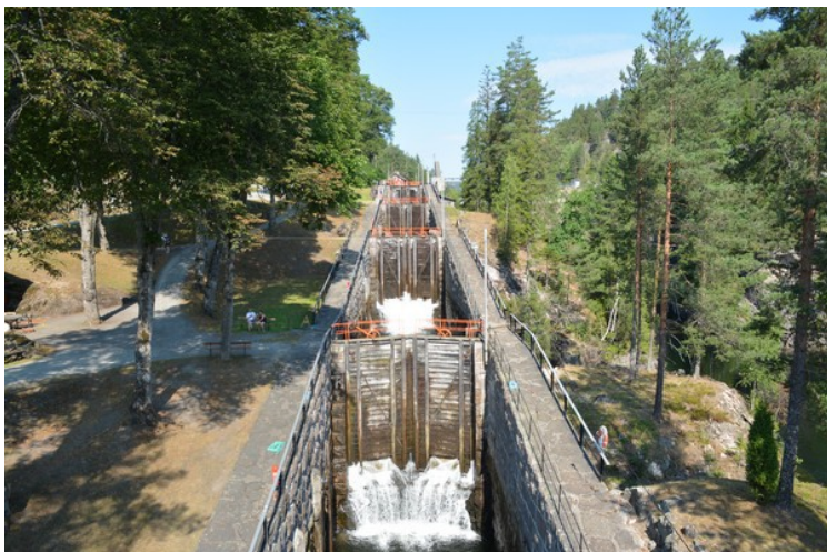
The flight of locks seen from below. There are 5 lock chambers here.
