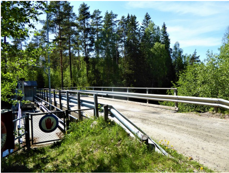
Here we have arrived at the Varald dam.
