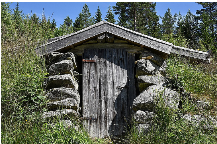
An earth cellar.
