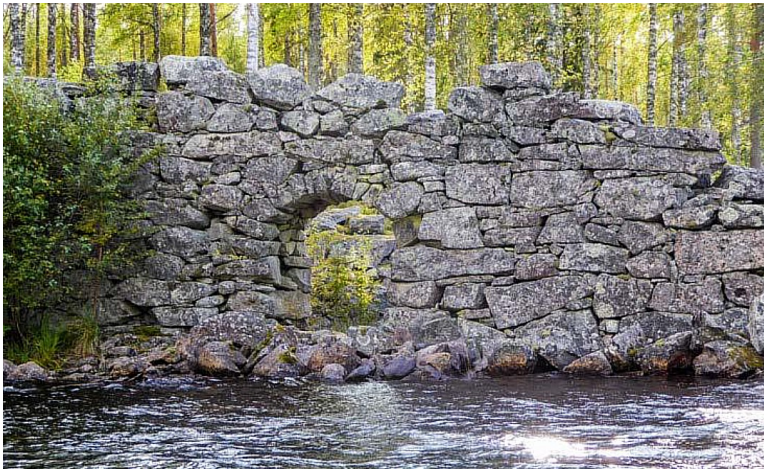
What is most visible here is the foundation wall of the sawmill.
