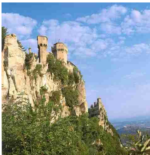
The towers seen from the other side. The third tower is the closest one.
