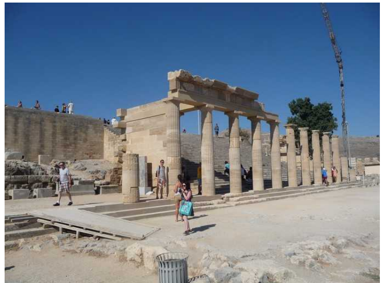
This is a Doric portico that is partially restored.
