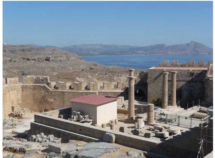
More restoration work in progress.
