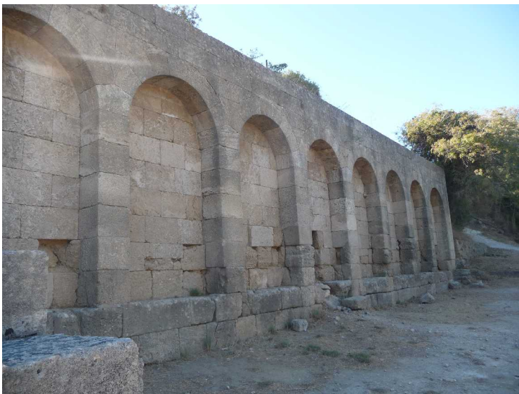
Here are some of the walls on the side of the theater. It is made a huge restoration work here.
