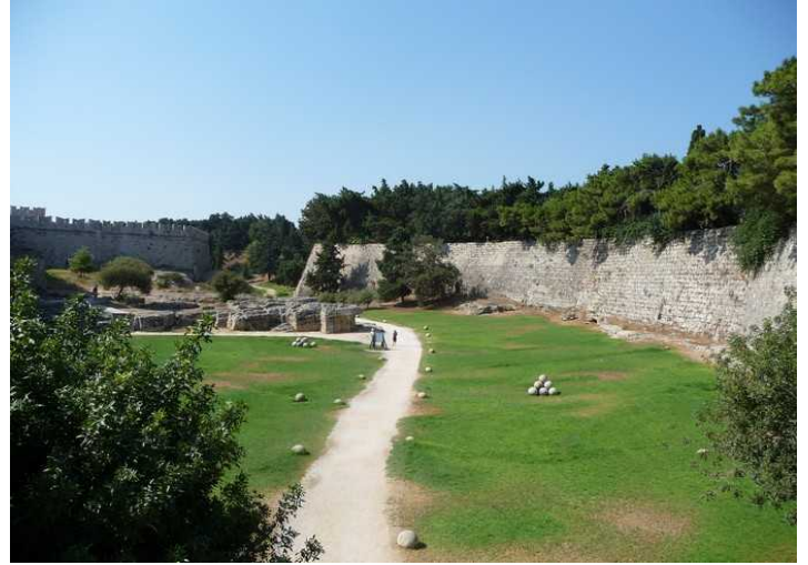
Here we see the area between the outer and inner ring wall, the moat. There are a lot of stone walls lying here. They were used in the mortars during the siege of the city.
