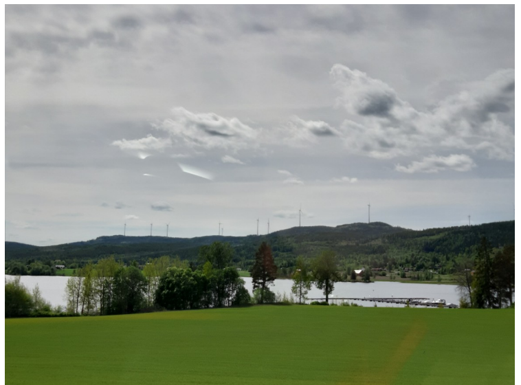
Here we see the wind turbines at Odal Wind Power Plant. It consists of consists of 23 wind turbines on Songkjølen and 11 on Engerfjellet.
