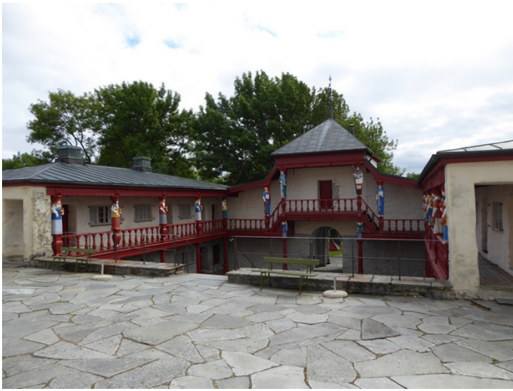
Up in the upper courtyard.
