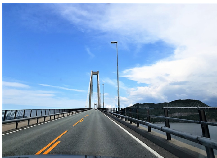
Here we are on Gjemnessund bridge . It goes across Gjemnessundet from Gjemnes on the mainland to Bergsøya.
