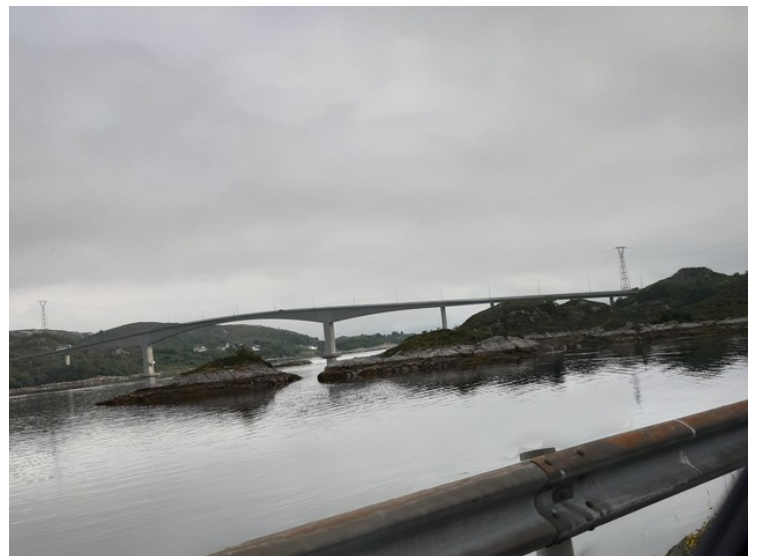
Here we drove over the Røysund bridge. From Nautøya we made a detour to Herøya.
