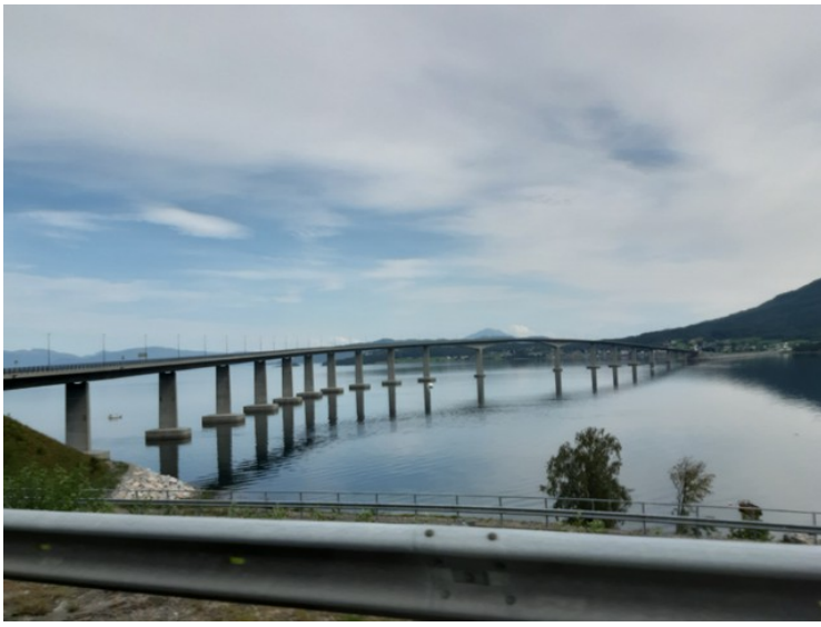
This is Tresfjord bridge that crosses Tresfjorden from Remmen to Vikebukta.
