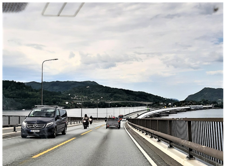
This is at the north end of the bridge where it comes to Flatøy.
