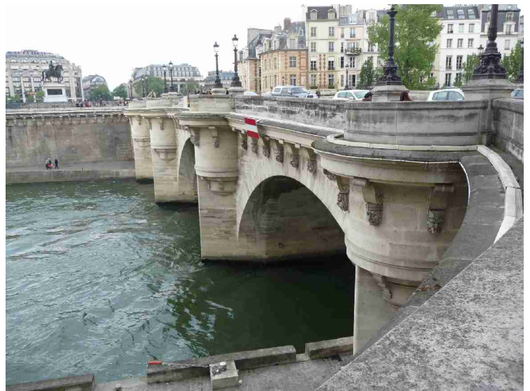
Pont Neuf, the oldest bridge in Paris. The bed stone was laid in 1578 by Henri 3. It is 275m long.
